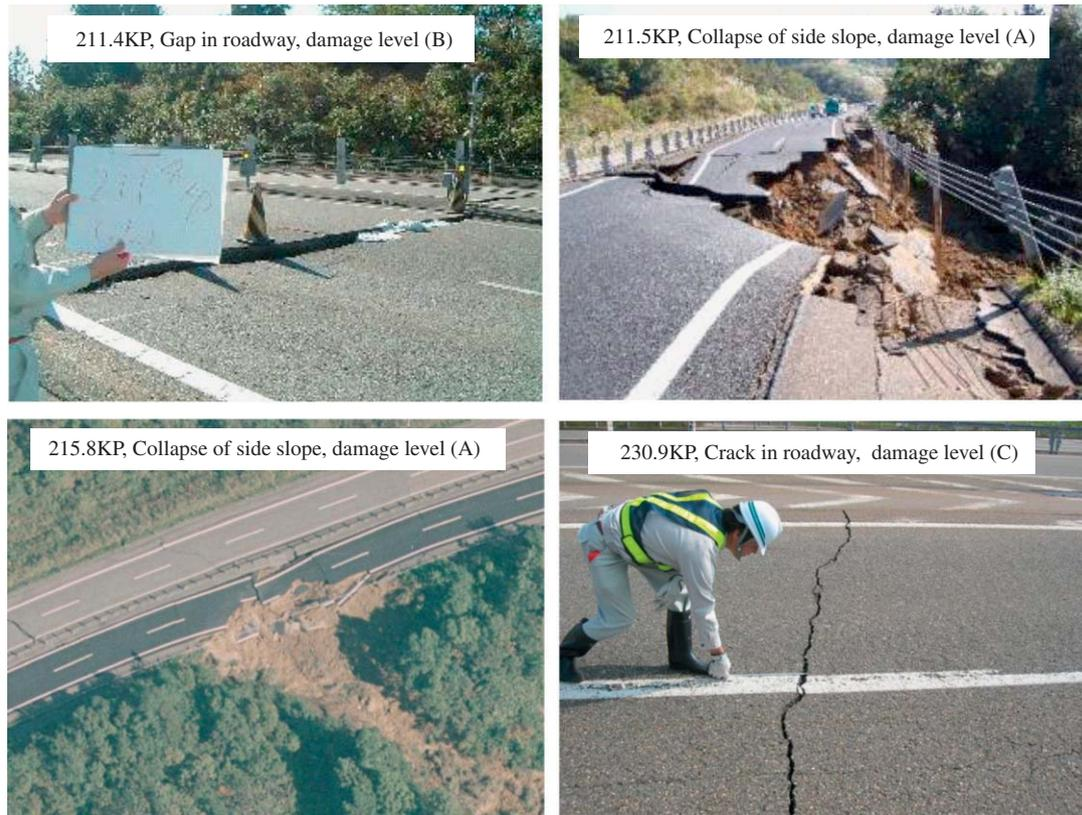
Fig. 1. Typical damage to expressway embankments after the 2004 Niigata Chuetsu earthquake.
