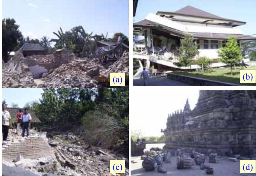
Figure 11. Typical damages seen in the field survey: (a) collapsed brick-masonry houses in a rural area, (b) a collapsed reinforced-concrete school building, (c) a large-scale landslide observed in a mountainous area, (d) stones fallen down from the towers in Prambanan temple compound.
