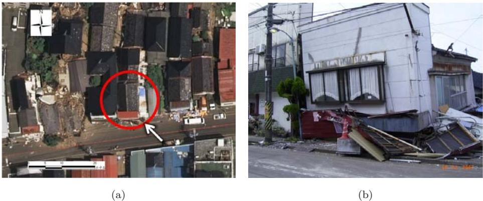
Fig. 1. Comparison between (a) the aerial image and (b) the field photo of the two-story building with the collapsed first story after the 2007 Niigata Chuetsu-oki earthquake.
