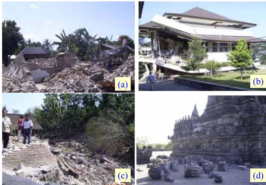
Figure 3. Typical damages seen in the field survey: (a) collapsed brick-masonry houses in a rural area, (b) a collapsed reinforced-concrete school building, (c) a large-scale landslide observed in a mountainous area, (d) stones fallen down from the towers in Prambanan temple compound.
