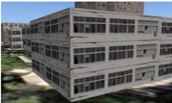
Figure 9. Cracked walls and windows
