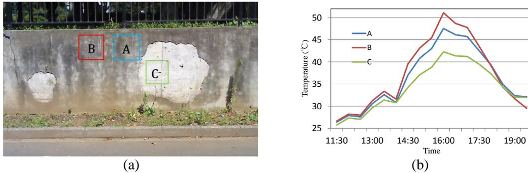
Figure 2. (a) The concrete retaining wall and the location of three target areas and (b) the temperature change in time at the three target areas.
