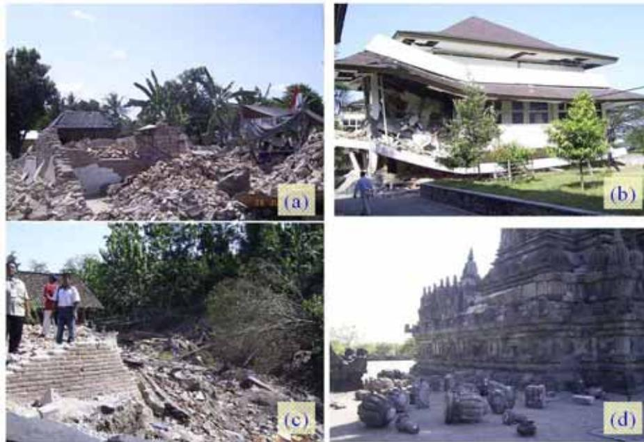
Figure 7. Typical damages seen in the field survey: (a) collapsed brick-masonry houses in a rural area, (b) a collapsed reinforced-concrete school building, (c) a large-scale landslide observed in a mountainous area, (d) stones fallen down from the towers in Prambanan temple compound.
