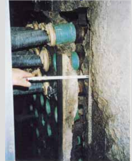
Pull out of cables at Manhole
