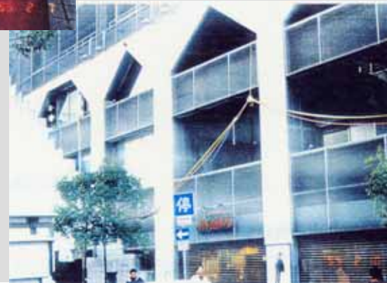
Temporary restoration using aerial cable
