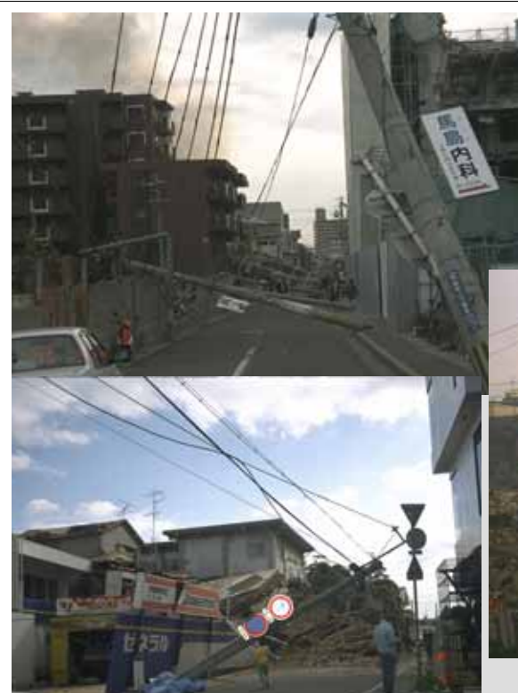
Electric Poles after the Kobe EQ
