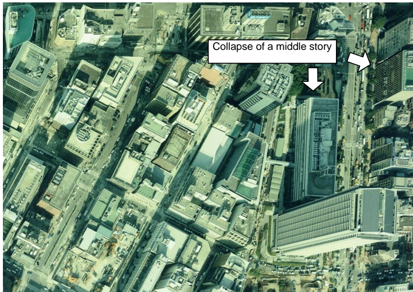
Photo 3: An example of aerial photographs for the non-wooden building area
