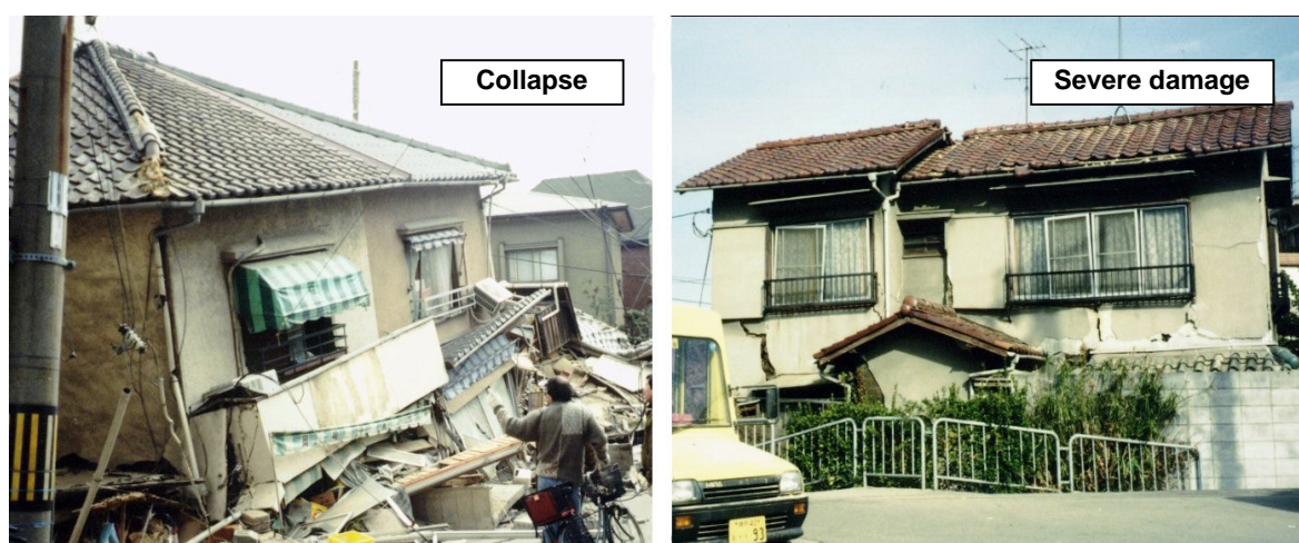
Photo 1: An example of ordinary “severely damaged” buildings and “collapsed” buildings
