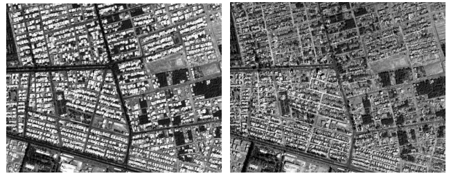
Figure 5. QuickBird images of the southeast part of Bam city taken before (left) and after (right) the Iran earthquake
