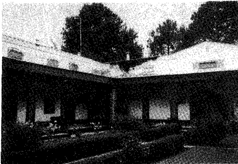
Photo 17 A damaged Pucca hotel in Saidu
