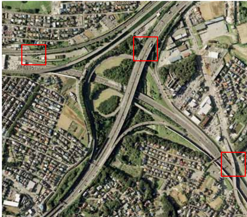
Figure 1: Aerial photograph of around Miyanogi junction, Chiba, Japan
