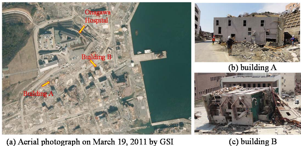
Figure 1 Aerial photograph of Onagawa Port area by the Geospatial Survey Institute (2011) on March 19, 2011 (a) and ground photos of overturned buildings by the tsunami taken on March 29, 2011 (b) & (c)
