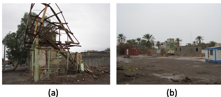
Figure 2. (a) Desolate building in the northeast of Bam and (b) bare land in the center of Bam
