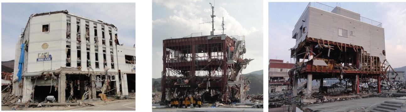
Figure 1. Typical tsunami damage to reinforced concrete and steel-frame buildings observed in our field survey after the 2011 Tohoku earthquake in Onagawa, Minami-Sanriku, and Ohtsuchi towns. The damage was concentrated to side-walls and lower stories of buildings.
