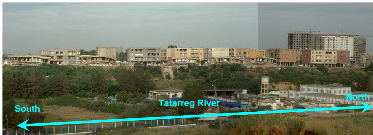
Figure 5. Photograph showing the heaviness of damage occurrence for buildings located on hill-tops in Zone 1A along Tatarreg river valley (see Figure 15). Also we can see that the buildings located very close to scarp edge were totally collapsed, while those located with distance away from scarp edge were partially collapsed or suffered extensive damage to structural elements, columns, and beams
