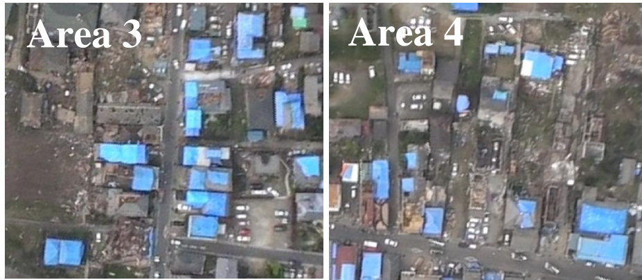
Figure 8 Target areas of heavy-damage in Figure 4.
