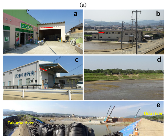
Fig. 3. (a) Mosaicked aerial photo of Mabi town, Kurashiki City (I), taken by GSI on July 9, 2018 [21]. Locations of bank failures and overflows are marked by the cross symbols. (b) Ground photos taken in the field survey on July 16, 2018, at the locations a–e in (a).
