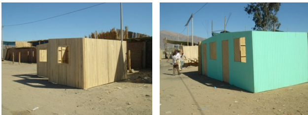
Fig. 8. Temporary house construction.
