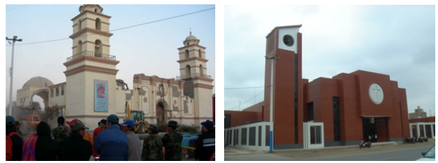
Fig. 2. Central San Clemente Cathedral of Pisco.
