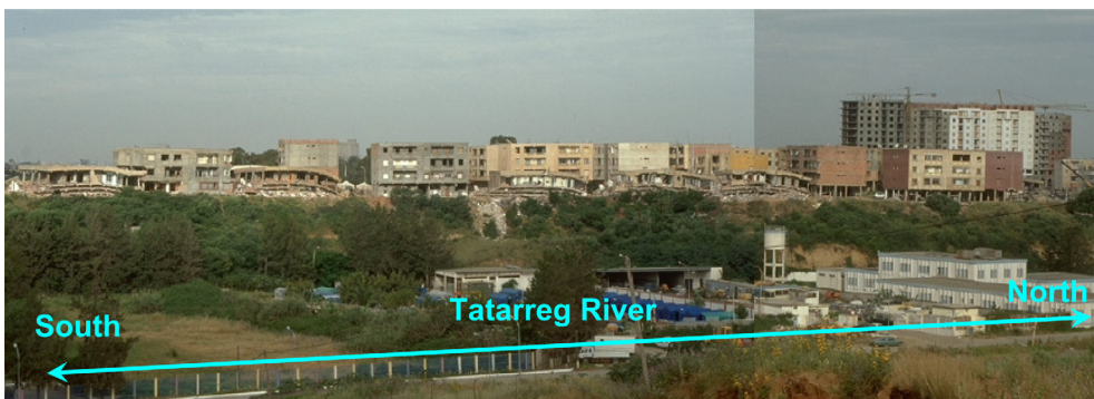
Figure 16. Photograph showing the damage to buildings located on hilltops in Zone 1A along Tatarreg River valley (see Figure 15). It can also be seen that the buildings located very close to the scarp edge collapsed totally, while those located some distance away from the scarp edge were only partially collapsed or suffered extensive damage to their structural elements, columns, and beams.
