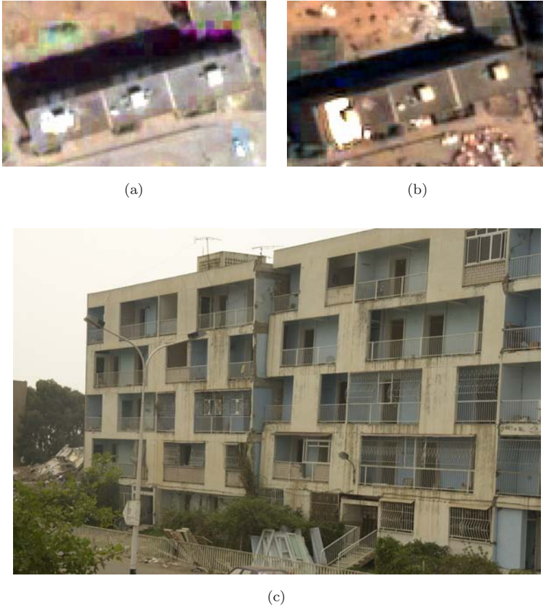
Fig. 10. Damage detection accuracy for a slightly tilted building: (a) the pre-event QuickBird image, (b) the post-event QuickBird image, and (c) a photograph from the ground.
