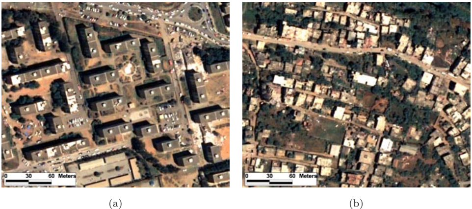
Fig. 2. Post-event images of Boumerdes city: (a) an area of modern medium- to high-rise constructions and (b) a densely built area mostly with low-rise constructions.
