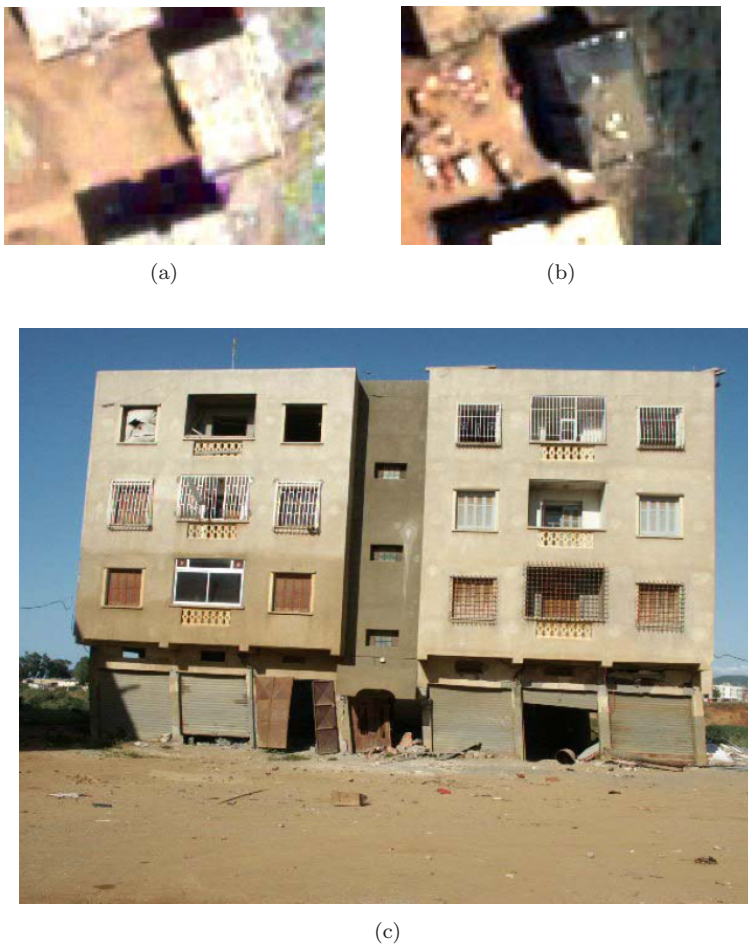
Fig. 9. A 4-story building that suffered from soft-story damage evaluated as Grade 4 from field survey; this structure was incorrectly judged as Grade 1-2 through visual detection from the QuickBird images: (a) the preevent QuickBird image, (b) the post-event QuickBird image, and (c) a photograph from the ground.
