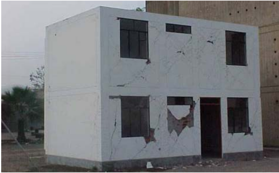
FIGURE 18: South wing of the house in final state
