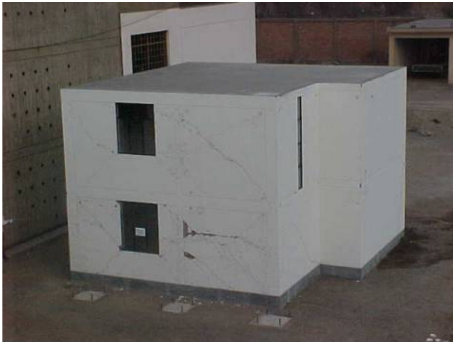
FIGURE 17: North wing of the house in final state
