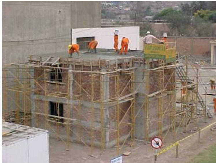
FIGURE 2: The building under construction
