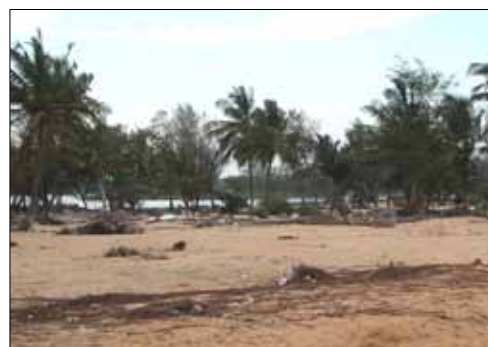
Washed away building
