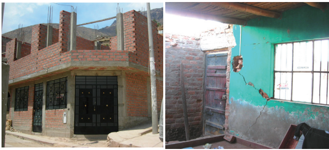
(a) Reinforced brick masonry (RM) (b) Unreinforced brick masonry (URM)
