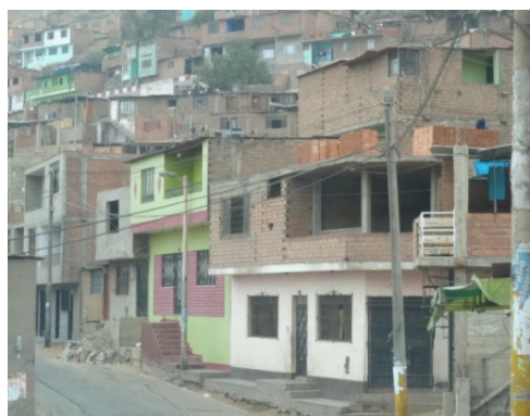
Fig. 1. Masonry houses in Lima.
