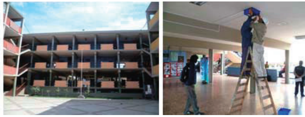
Fig. 6. Seismic monitoring system of buildings in Lima.
