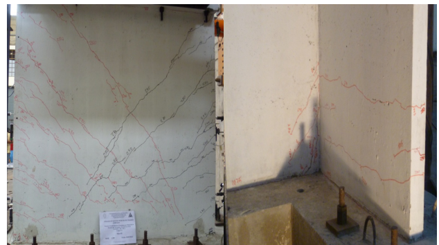
Fig. 18. Final stage of one-plane wall and H-shaped walls.
