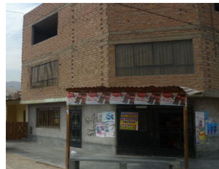
Fig. 2. Building with URM wall.
