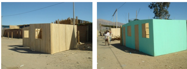
Fig. 8. Temporary house construction.
