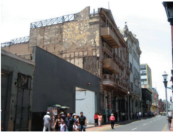
Fig. 5. Typical quincha construction.
