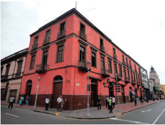
Fig. 8. Typical quincha construction for measurements.
