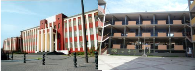
Figure 3 Central Building and G2 bldg block (North view) at Civil Engineering Faculty at UNI
