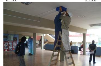
Figures 8 Central Block in G2 FIC and setting of sensors to the ceiling (below)
