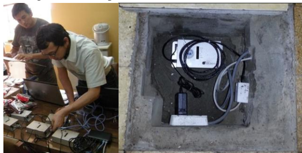
Figure 2 Network setting test and final placement of sensor at basement level in UNI Central Building
