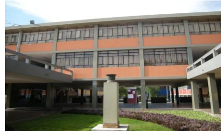
Figure 6 Location of Central Block G2 in FIC and South side view of building
