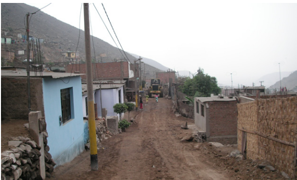
Figure 2 Photograph of the condition of the buildings on the hillsides.
