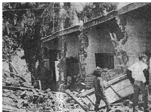
Figure 1: Destruction in La Molina area 1966 quake
