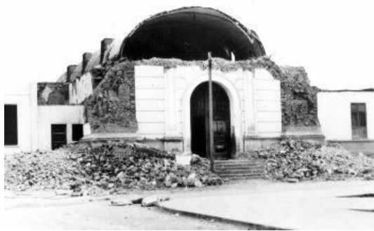
Figure 2: Collapse church's roof -1974 quake
