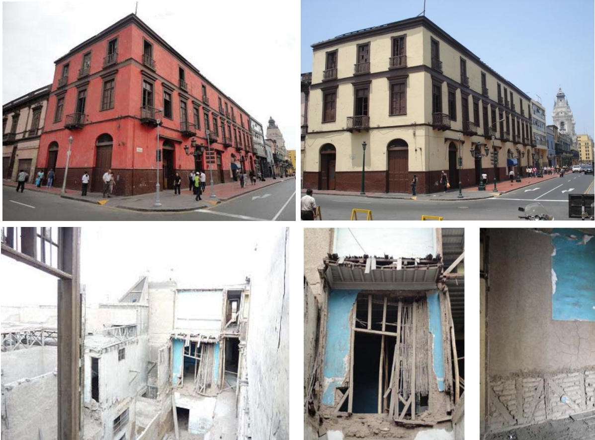
Figure 2. Typical adobe-quincha construction and structural condition details
