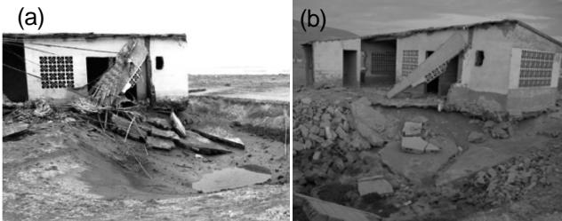
Figure 3 Damaged house and destruction of the foundation in (a) 2001 (Dengler, 2001) and (b) 2010
