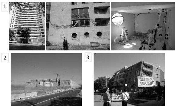
Figure 2 Survey route and field photos in Santiago—April 2, 2010
