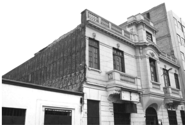
Figure 4 Typical quinchá wall at Lima centre
