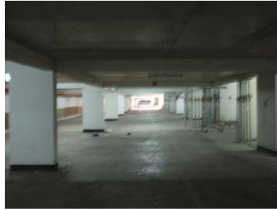
Photo 2 Underground parking lot
