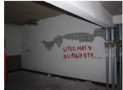
Photo 3 Shear wall on the first basement
