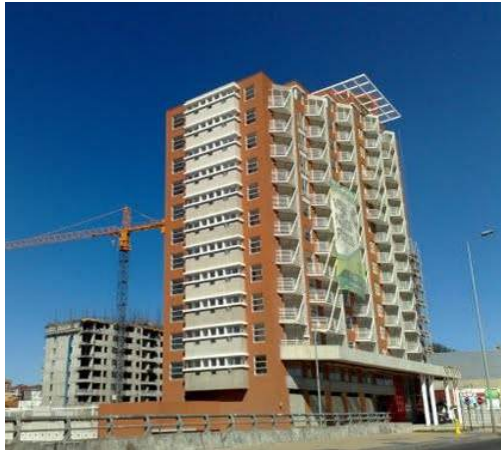
Photo 6 Photo of the building before collapsed (excerpted from the Web Page)
