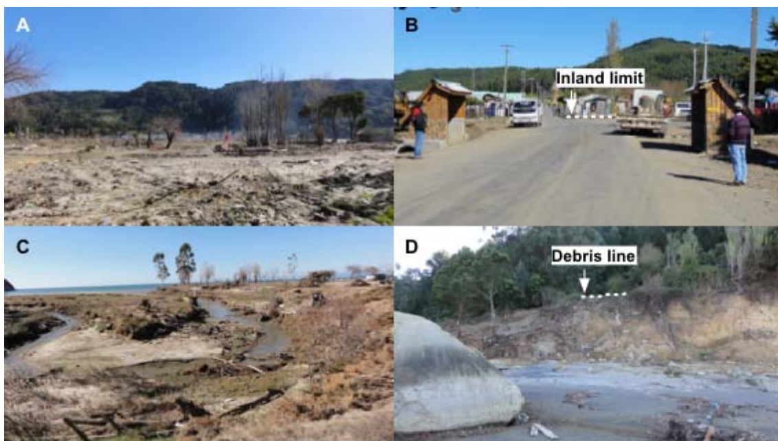
Fig. 13 Ground photos from Llico. A : Completely devastated village. In the village, there were around 60 houses before tsunami. Almost all the houses were washed-away. B : Inland limit of tsunami inundation that is approximately 400 m from the shoreline. C : Tsunami run-up along the river. D : Tsunami debris line above 14.8 m pre-tsunami sea level.
