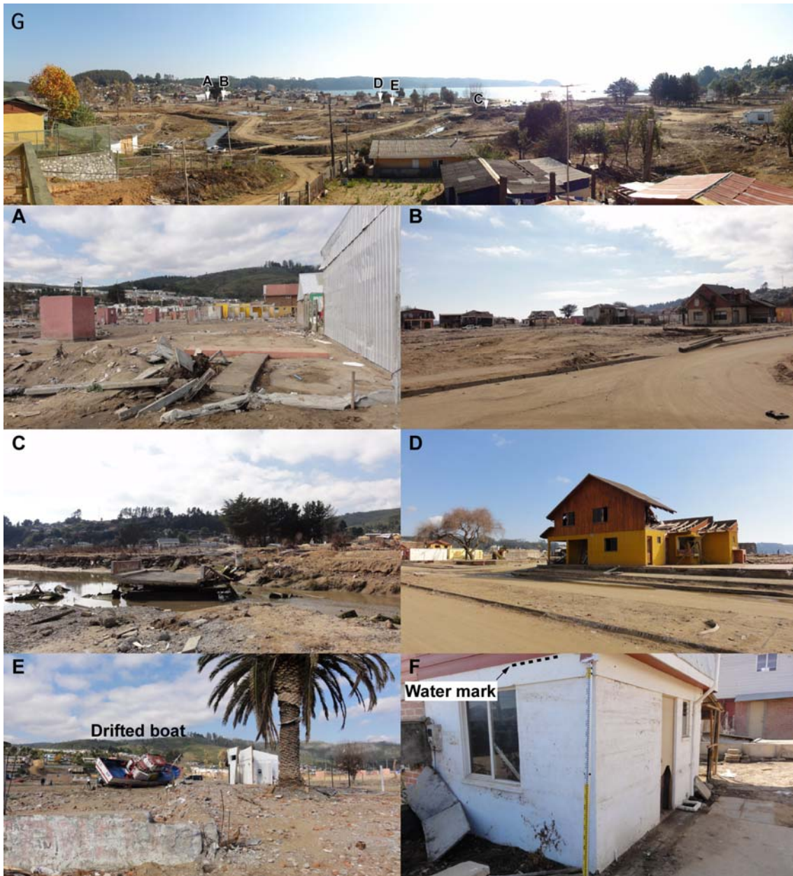
Fig. 16 Ground photos from Dichato. A and B : Most devastated area. Only the unit of bathroom is remained. C : Damage on a bridge and erosion by tsunami inundation. D: Withstanding house, but significant damage. E : Drifted boat. F : Watermark on the house (approximately 2 m of flow depth). G : Panoramic view of the town of Dichato.
