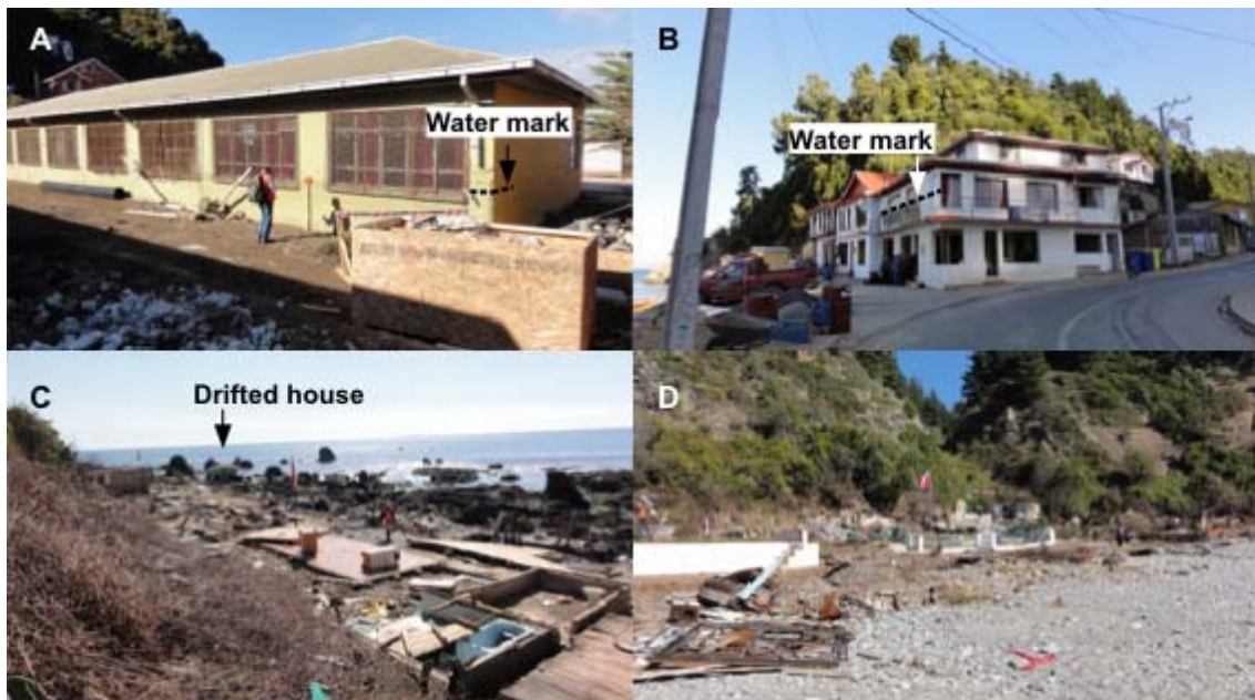
Fig. 11 Ground photos from Tumbes (A, B) and from Puerto Ingles (C, D). A : Watermark on school building. B : Watermark on the house of Tumbes, C and D : Completely devastated village of Puerto Ingles.
