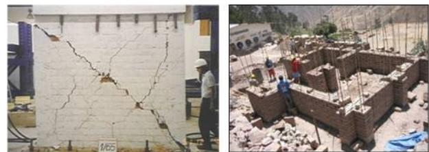
Fig. 7: Structural testing (left) and construction site of reinforced masonry house (right)
