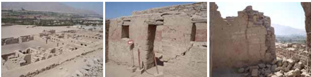
Figure 8: Some views of Tambo Colorado effected by earthquake motion
