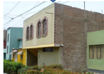
Reinforced or confined masonry with rigid slabs (M3, M4)
