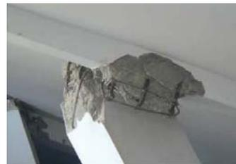
Damage to reinforced concrete building with insufficient seismic resistance in Pisco city
