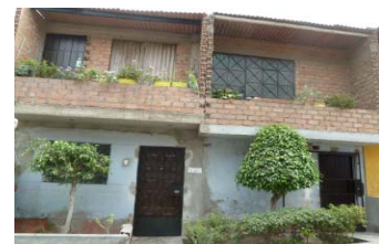
Non-engineered masonry (M1) or Reinforced or confined masonry with flexible slabs (M2)
