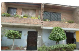
Non-engineered masonry (M1) or Reinforced or confined masonry with flexible slabs (M2)
