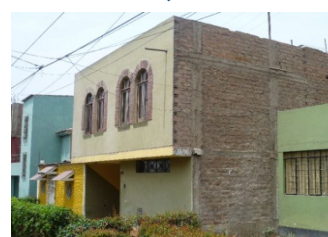
Reinforced or confined masonry with rigid slabs (M3, M4)
