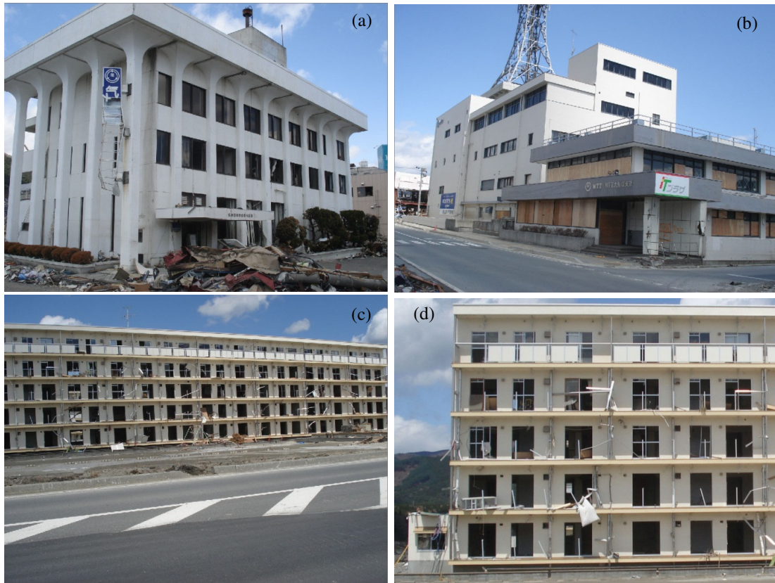
Figure 5: RC buildings after tsunami attack
