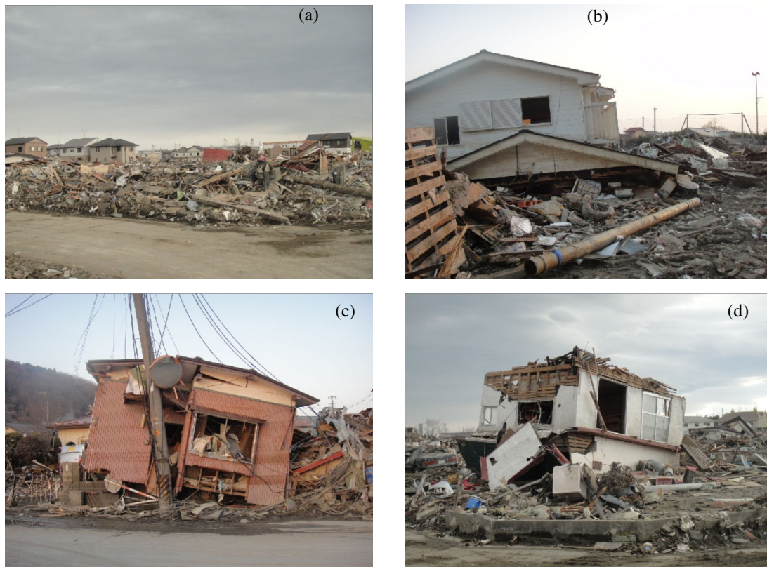
Figure 3: Damages on wooden houses
