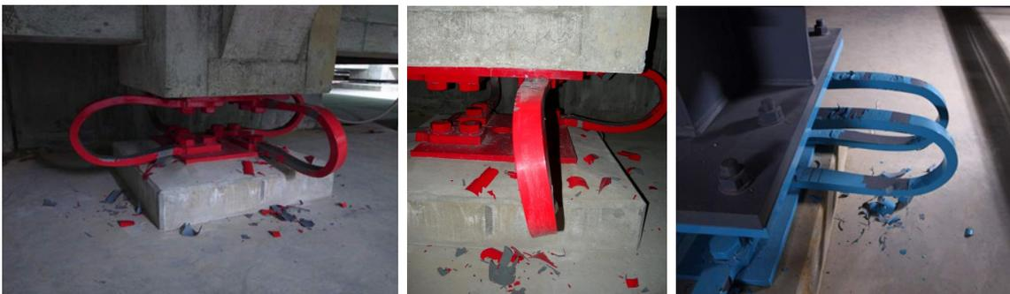
**Figure 9.** Peeling off of paint of steel dampers
