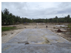
Damage in Muntei
