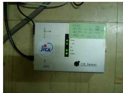
2nd Floor: office room
