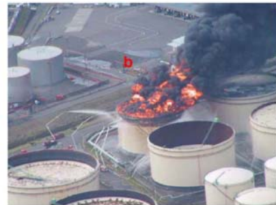
Fig. 3 Open-top fire in a naphtha tank (tank B, photograph courtesy of Sapporo Fire Bureau)
