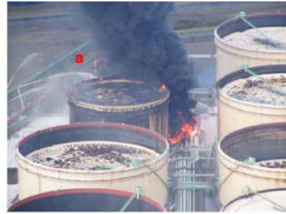
Fig. 2 Ring fire in a crude oil tank (tank A photograph courtesy of Sapporo Fire Bureau)
